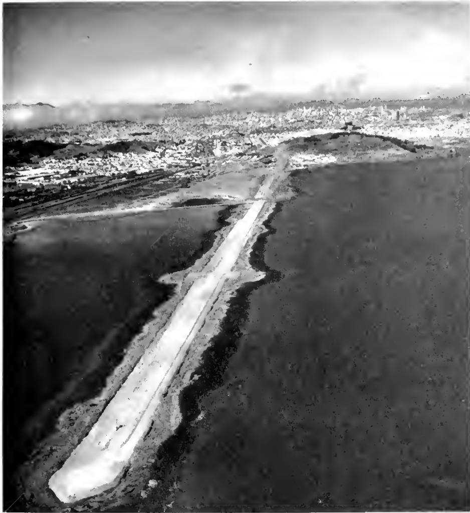
Fill for open water section of Bayshore Freeway across Candlestick Cove. Widening at center of picture is location where reinforced concrete box culverts will be constructed to equalize water level.
